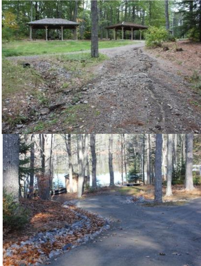
Figure 1. Before and after photos of camp road.
