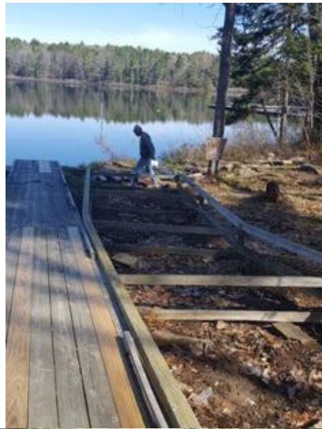
Figure 3. Boat access/storage site with bare soils and runoff in 2016. In 2017, road resurfaced; ditch/plunge pool installed and boats stored upland from shore.
