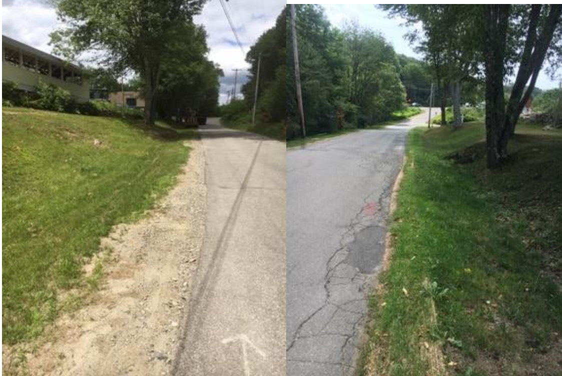
Figure 7. Road shoulder erosion, before and after stabilization and seeding.
