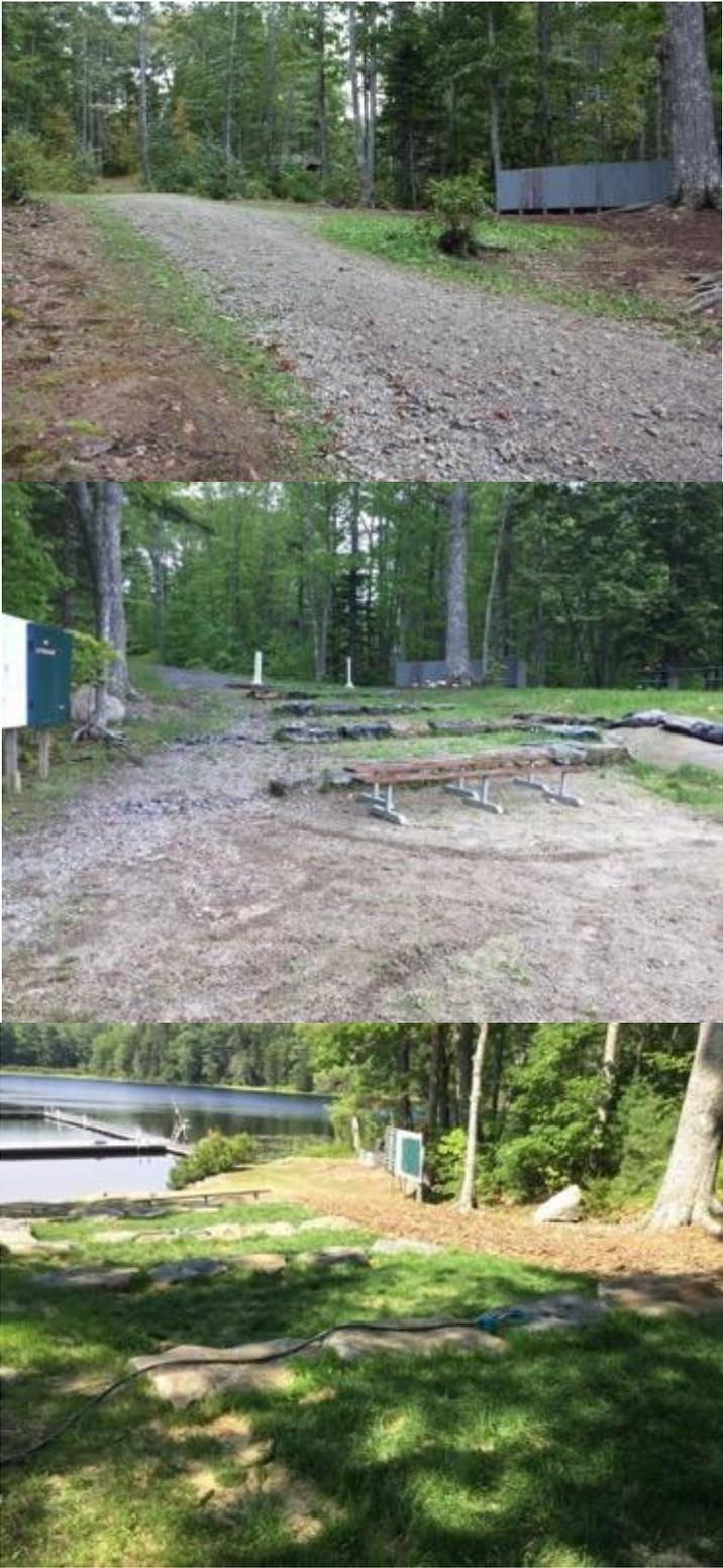
Figure 3. Boat access/storage site with bare soils and runoff in 2016. In 2017, road resurfaced; ditch/plunge pool installed and boats stored upland from shore.
