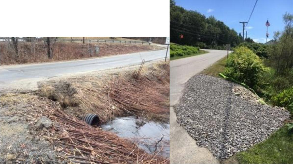
Figure 7. Road shoulder erosion, before and after stabilization and seeding.
