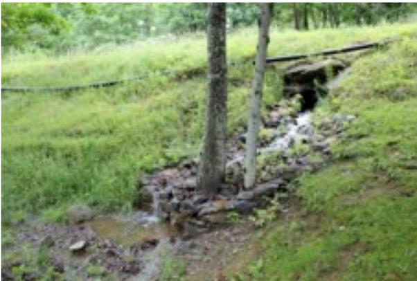
This unstable, poorly designed and maintained culvert has caused significant erosion of a residential property on Knickerbocker Lake. Culvert replacement with proper design to slow and intercept flows is needed.
