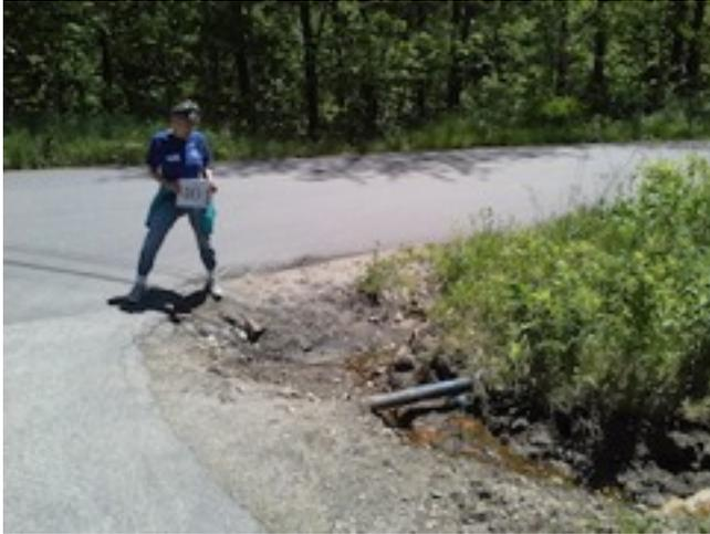
Erosion around culverts and roadway ditches was seen at several road sites during the survey.
