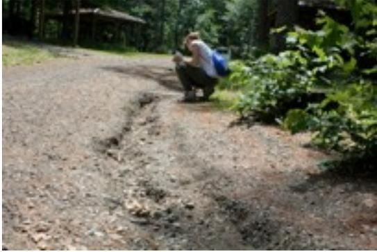
Erosion of this private road on Knickerbocker Lake has resulted in sediments and phosphorus entering the lake.
